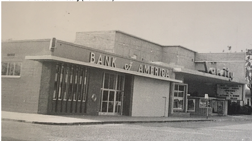
Figure 2. Subject building photographed in 1953 during original occupancy by Bank of America. This photograph shows the building's original appearance, prior to 1972 alterations. (Lofland and Haig, Images of America: Davis California 1910s-1940s , photograph credit to John W. Brinley)
